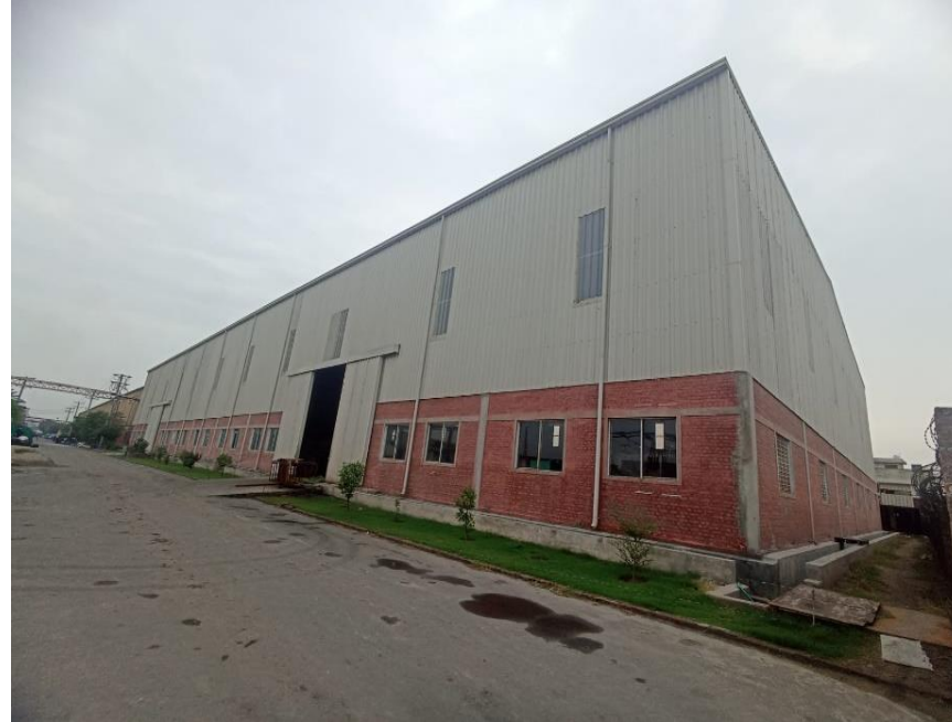
Building for Calendar department PKR 173.9 Million
